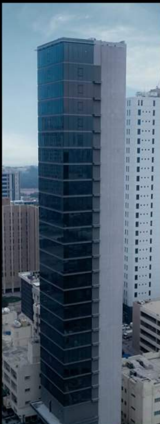
YJM Medical center Tower | KUWAIT-2019
